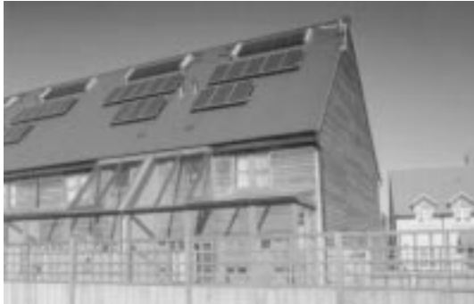
Low energy housing, Cambourne - in denial of its heritage aping neighbours
