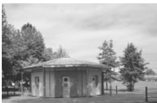
Gonville Place Lavatories
